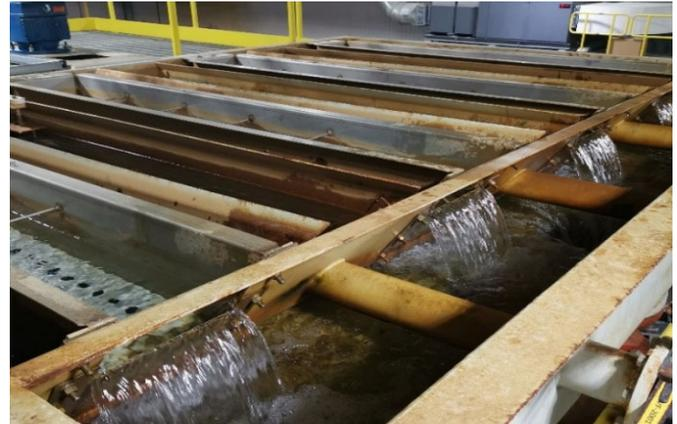
**Photo 3.50 Treated water at the outlet to the lamellar clarifier**
