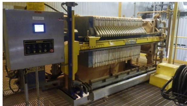
**Photo 3.53 Sewage treatment sludge press machine at mine wastewater treatment plant (MWWTP)**
