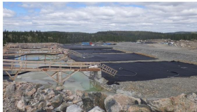
**Photo 3.51 Modular treatment plant with Geotube® filter bags**
