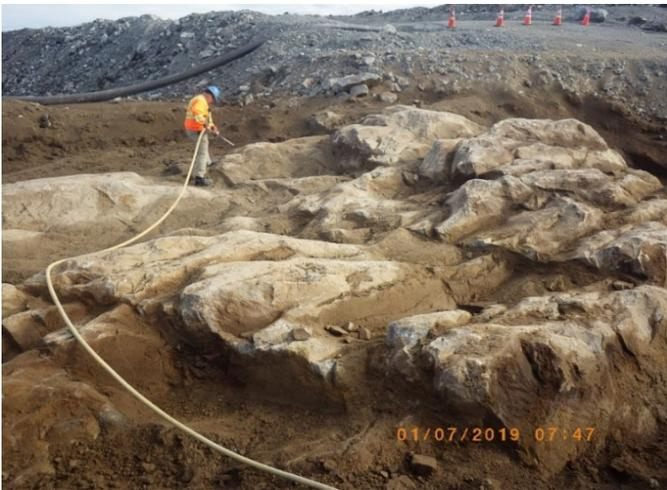
**Photo 3.57** Compressed-air cleaning of bedrock foundation, which had been stripped using an excavator.
