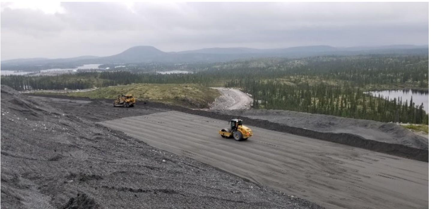
**Photo 3.59** Placement and compacting of coarse PK to raise the layer downstream of the center line.
