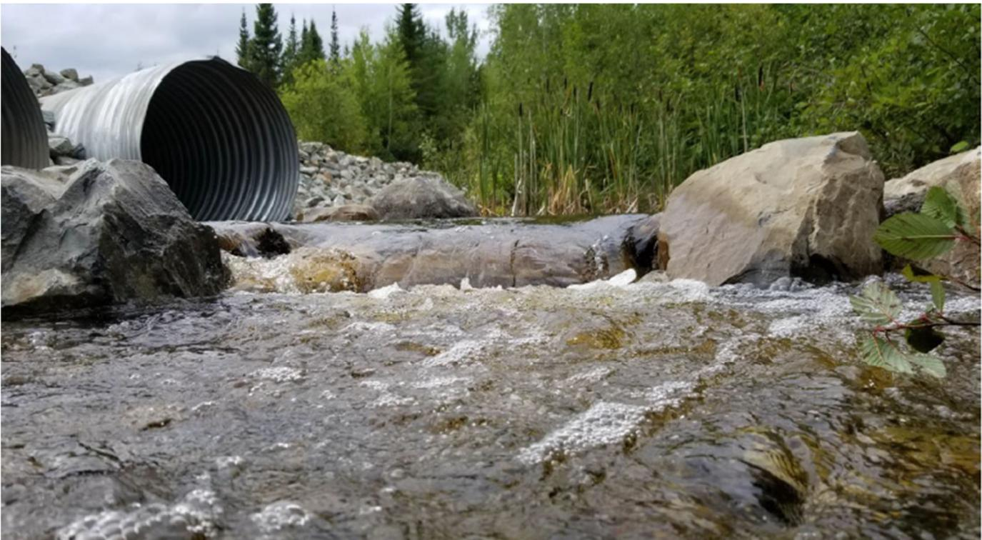
Photo 3.34 Riffle developed downstream of culverts
